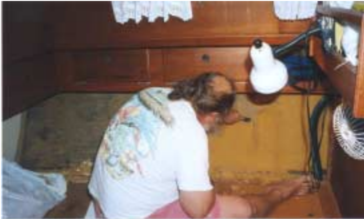
Scraping out the old foam
