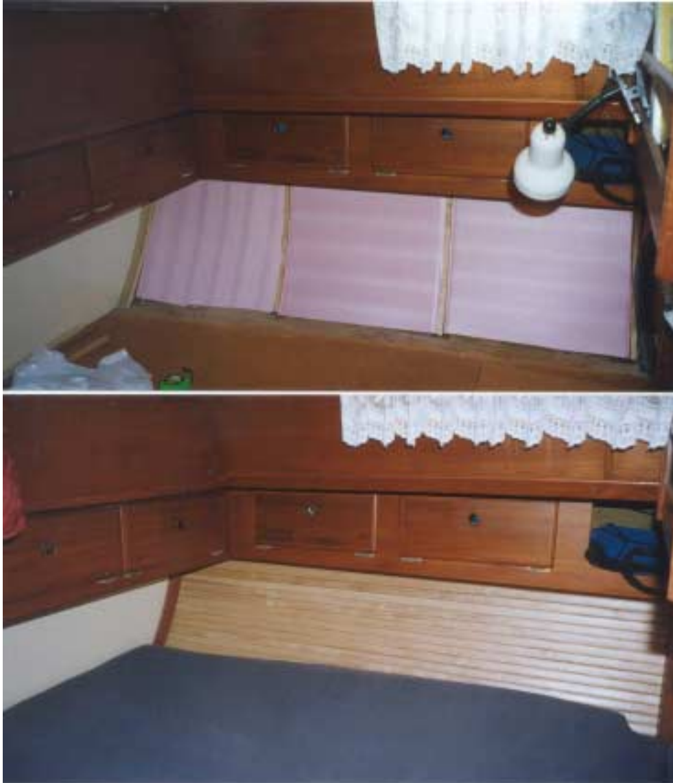
Foam insulation and finished product.
