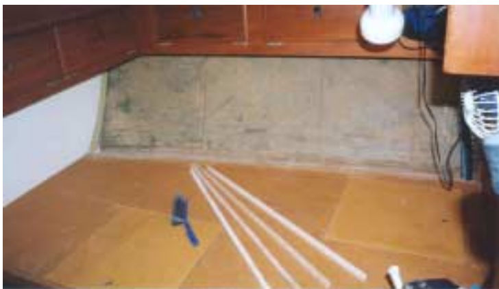
Cleaned and marked for furring strips.
