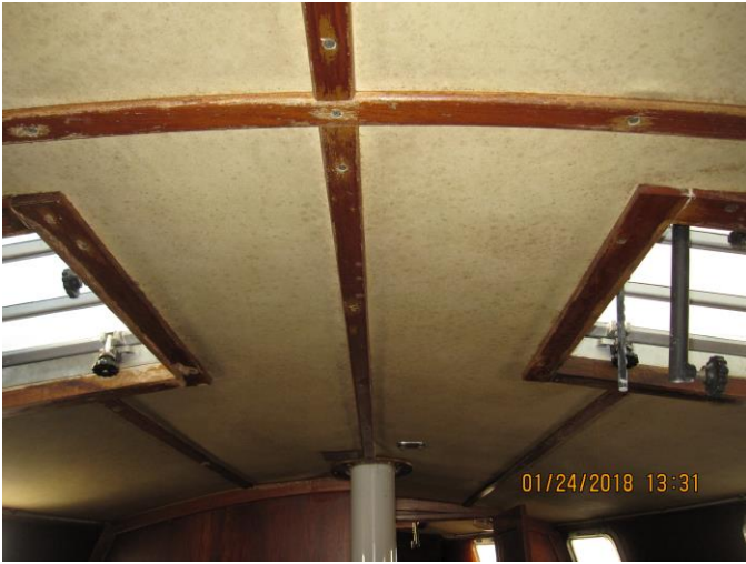
Mildew on vinyl panelboard headliner
