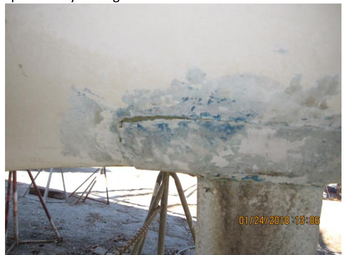
Cosmetic fairing cracking around propshaft strut
