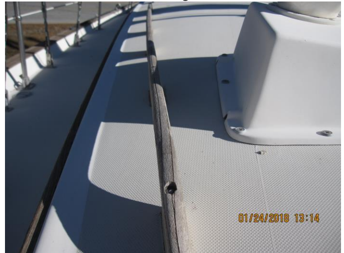
Hand rails thinned, fasteners exposed
